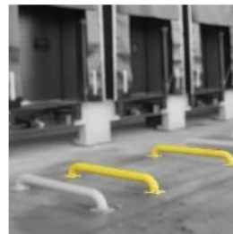
Wheel guide To center the truck Ø139 L=2000mm
