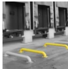
Wheel guide To center the truck
